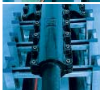
All fixed. Anchoring clamps for fixing cables against longitudinal stretching in steep terrain.
