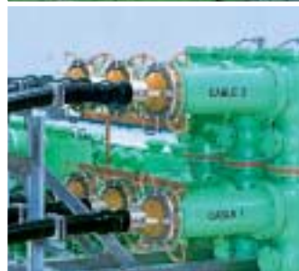
TFF 1.275-11 Sealing ends for parallel cable insertion in SF6 switchgear with short-circuit resistant supports.
