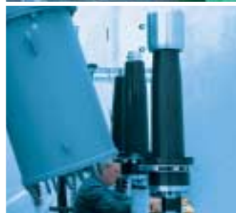
TT 1.170-11 Sealing end for single-pole insertion in transformer entrance box.
