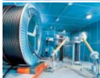
Routine testing. Screened and protected room for routine testing, guaranteeing the highest quality standard of the insulation system.
