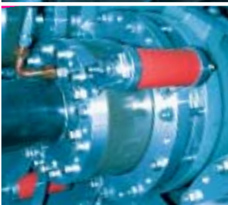
Safely protected. Sheath overvoltage arrestors across the isolated part of the SF6 sealing end protect the outer sheath from surge voltages.
