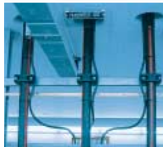
Fastening in basement. Alignment and fastening of high-voltage single-core cables in cable basement.
